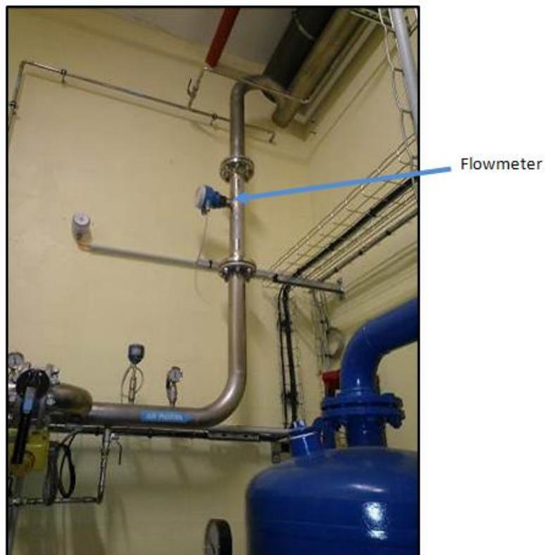
Fig. 4. Compressed air flowmeter location
