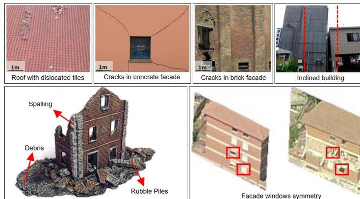
**Fig. 7. Examples of remote sensing [40]**
